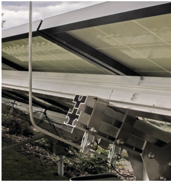
Figure 2 Lightning protection by means of DEHNiso spacers
