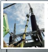
The PHE4 voltage detector with sufficiently long insulating stick is ideally suited for use in **out-door switching stations**.
