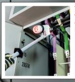
The compact design of the PHE4 voltage detector is beneficial in **electrical switchgear assemblies**.
