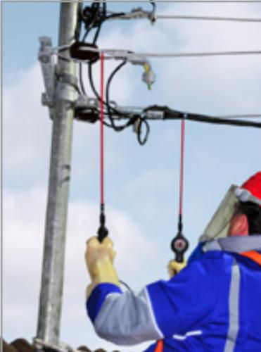
With screwed-on extensions, it is possible to work at a safe distance from open circuits and current rails in switchgear.
